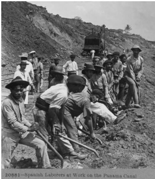
Figure 4. Everett Collection, Inc. Alamy, Canal Construction 1909. 23
